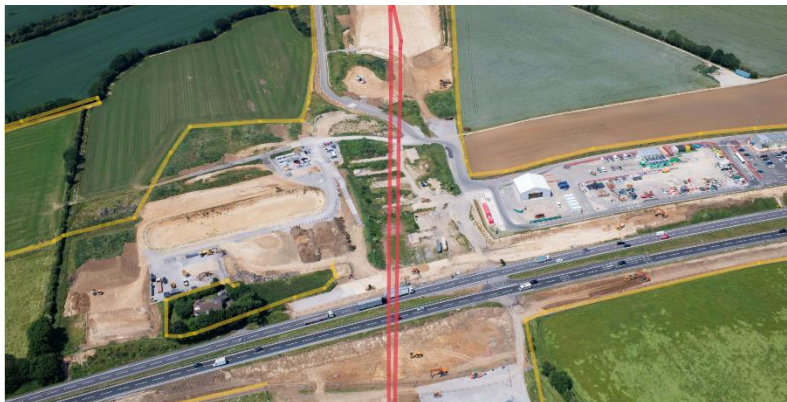
Construction of temporary diversion route
