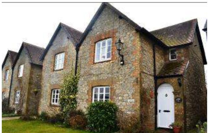
Figure 45: Example of limestone property with brick lintels and quoins.
