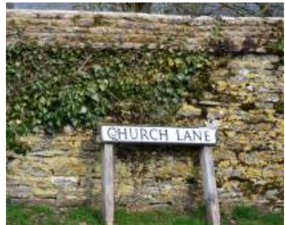
Figure 41: Example of historic boundary wall that runs along Church Lane.
