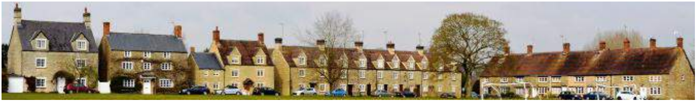
Figure 46: View across the green illustrating the uniformity of chimney stacks in the conservation area.
