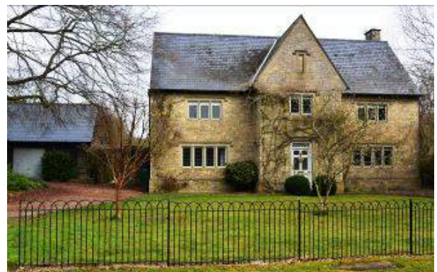
Figure 16: An example of a larger scale property down Church Lane a good example of a contemporary building utilising local materials and similar vernacular detailing.
