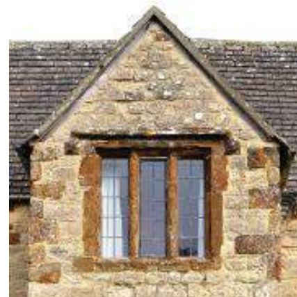
Figure 52: Seventeenth century stone mullions with hood and stop moulding.
