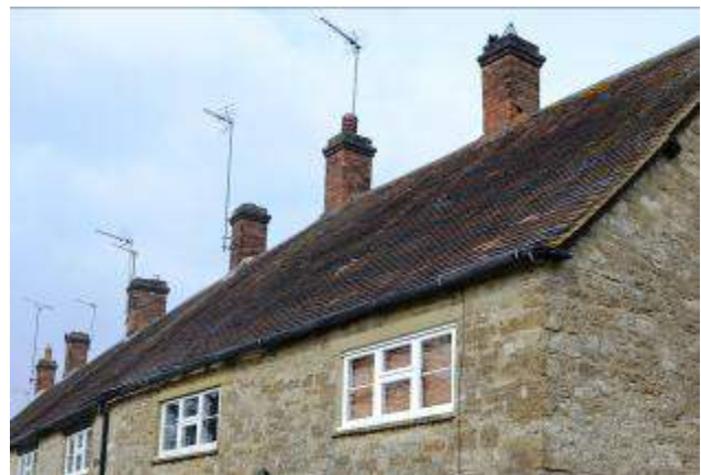
Figure 26: Antennae on chimney pots.
