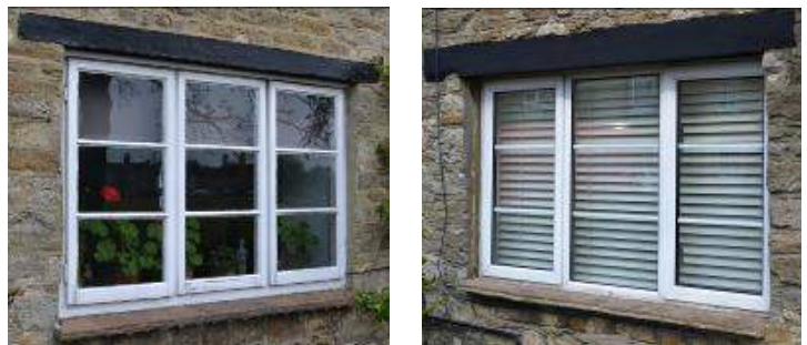
Figure 51: Example of wooden glazing bars (left) and PVCu alternative (right).
