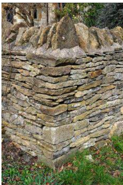
Figure 44: Example of dry limestone wall with cock and hen coping.
