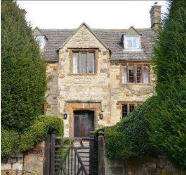
Figure 35: Seventeenth century Manor House with ironstone detailing, hood mouldings and stone mullions.
