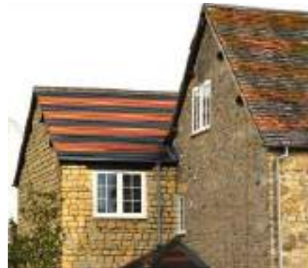
Figure 47: Alternating red and black tiling prevalent throughout the area.
