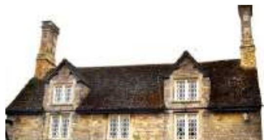
Figure 49: Distinctive stone chimney stacks on the Red Lion Pub.
