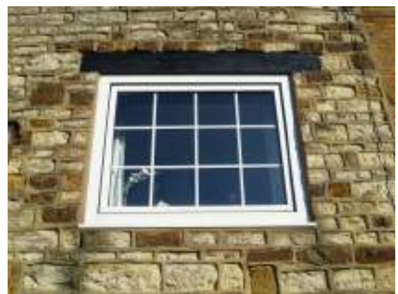
Figure 62: (above) shows a more traditional timber casement window in contrast to the modern PVCu window seen (below)
