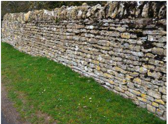
Figure 13: Historic stone boundary wall which can be seen along Church Lane.
