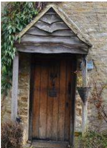
Figure 57: Example of a timber porch.
