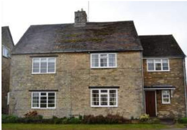
Figure 43: Example of limestone coursing within the Conservation Area.
