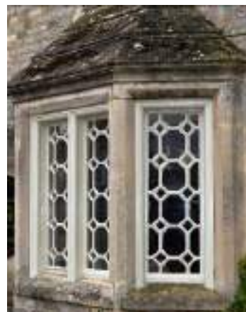
Figure 53: Cast iron windows with octagonal shaped panes on The Red Lion.
