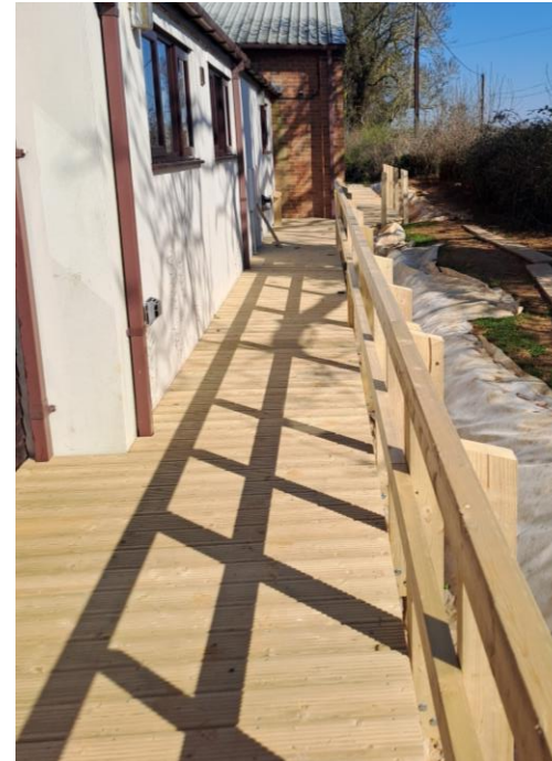
Volunteers built ramped access to Chipping Warden Village Hall
