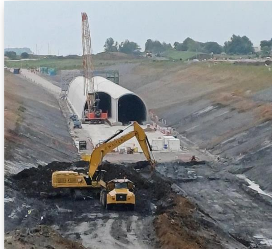
Greatworth – earthworks progress and waterproofing gantry in place
