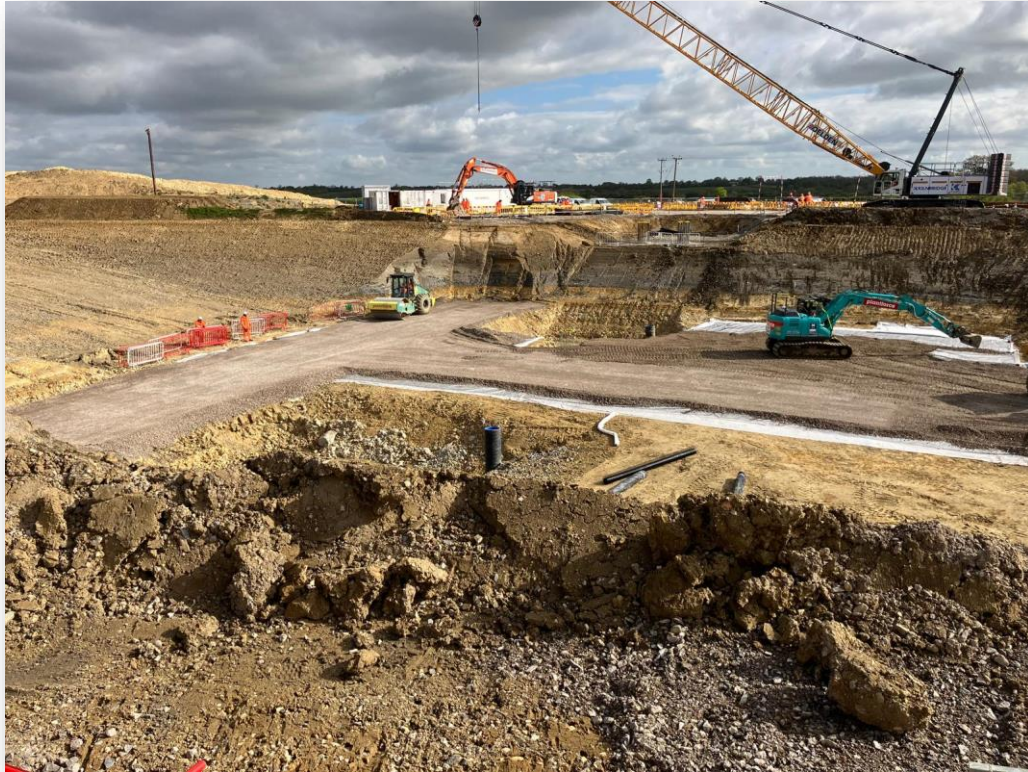
AX18 Piling complete – Preparation for the concrete
