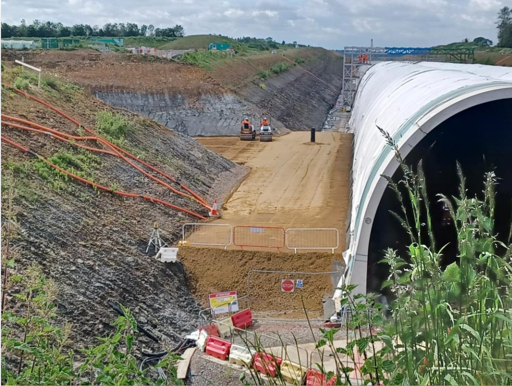
Chipping Warden – backfill has begun
