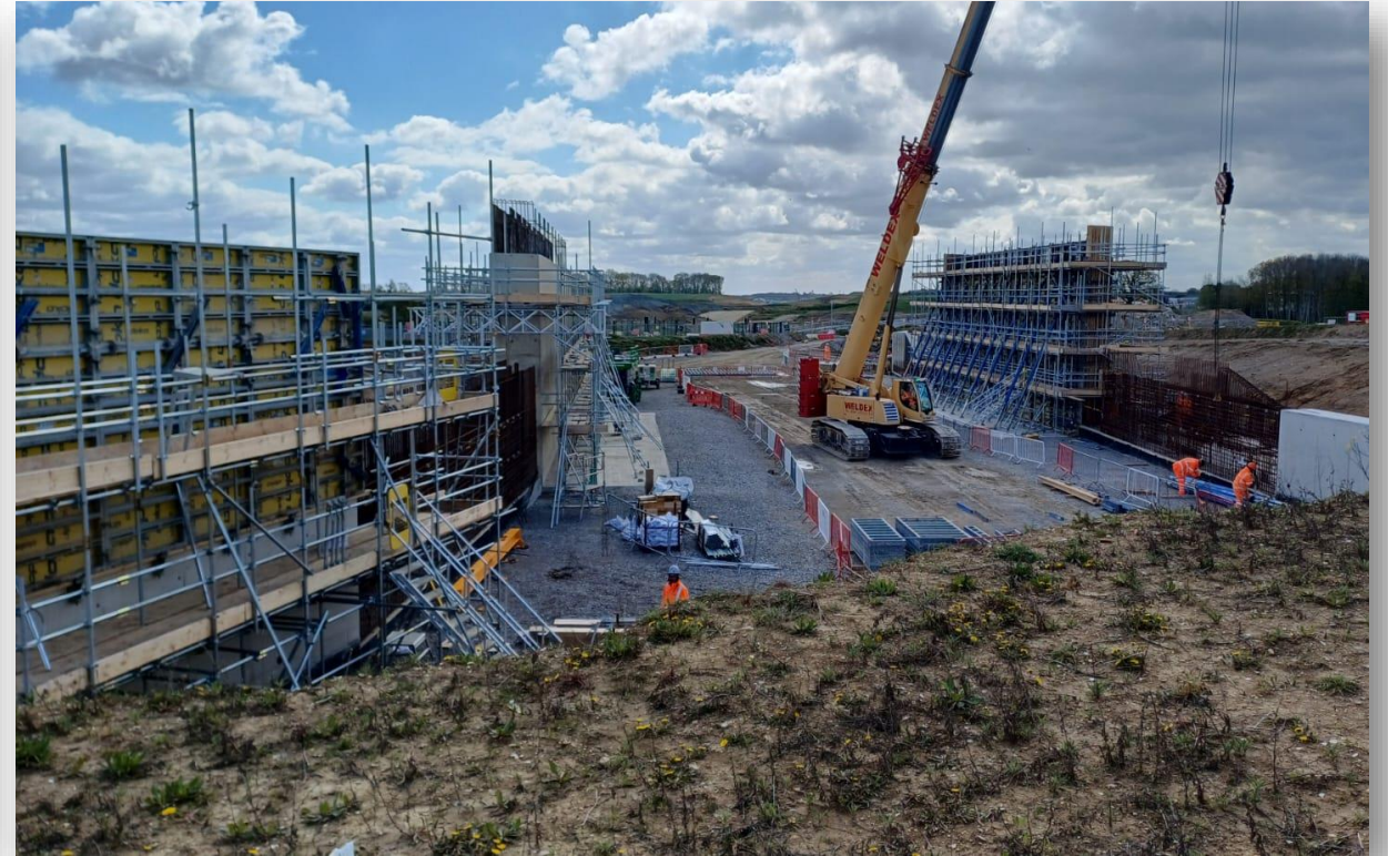
Wing wall construction
